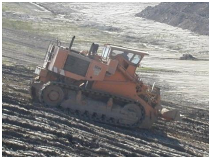
SR 264 at scraping
