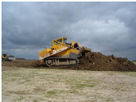
Dumping of topsoil on a distance of 100m
