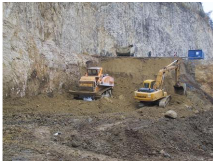
Digger in cooperation with Scrapedozer
