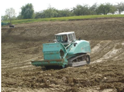
Dismantling and loading
